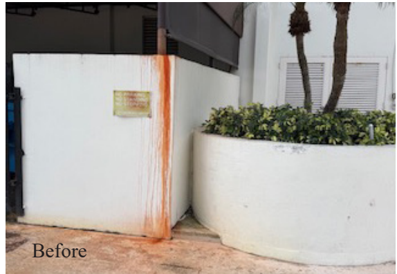
Pressure clean and paint walkway by west end building C and replace canopy
