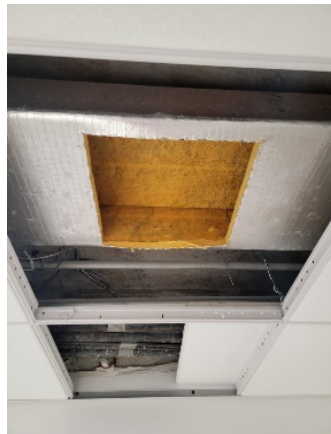
New a/c diffuser & connection
