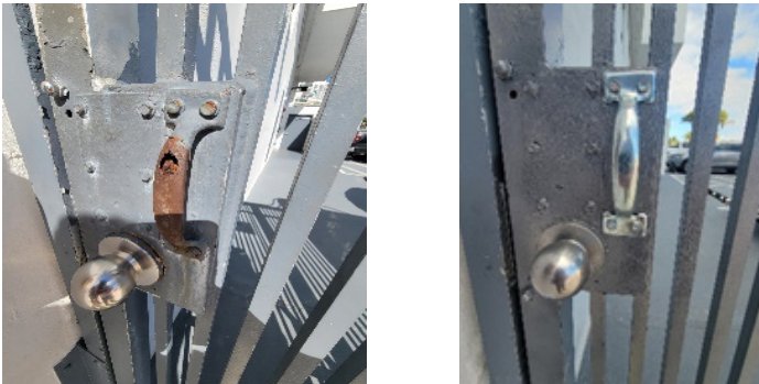
corroded handle
