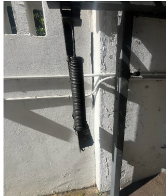
Broken gate bracket
