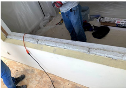
Pictures of existing wood bucks and concrete sill.
