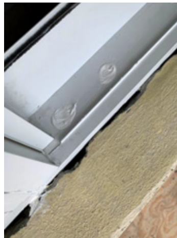
8. Pump Dow 795 into punched sill tap-con holes to protect concrete/ from water intrusion. Finish by sealing screw heads.
