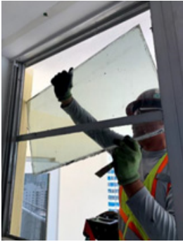
5. Remove glass panels from existing system.
