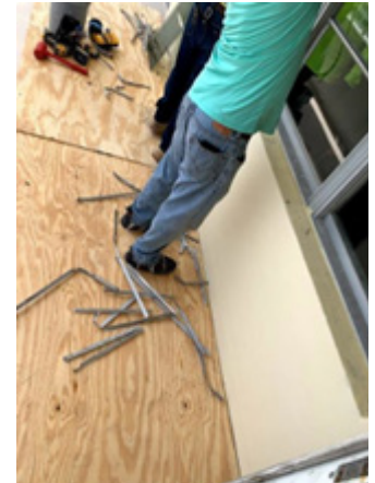
2. Protect exterior waterproofing with plywood (where balconies apply)
