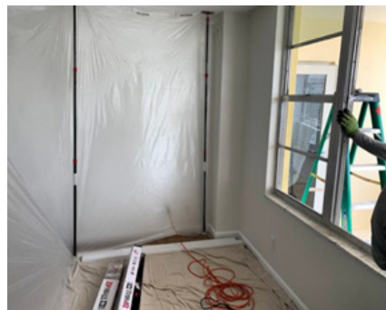
3. Install dust walls in order to protect units from dust.
