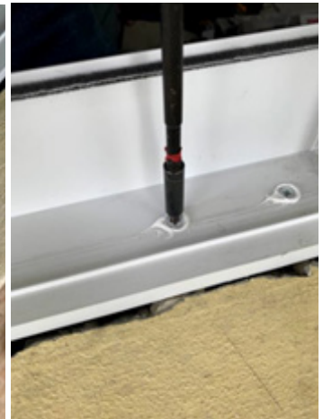
8. Pump Dow 795 into punched sill tap-con holes to protect concrete/ from water intrusion. Finish by sealing screw heads.
