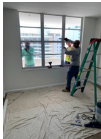
1. Protect interior flooring with drop cloths to catch debris from demolition
