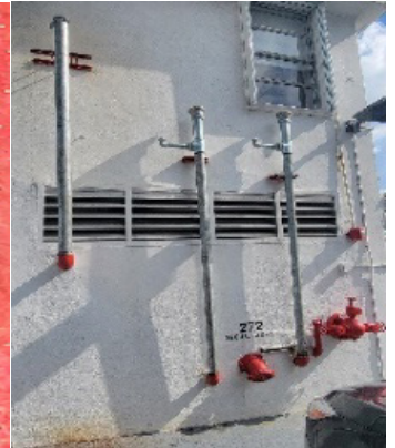
three new pipes
