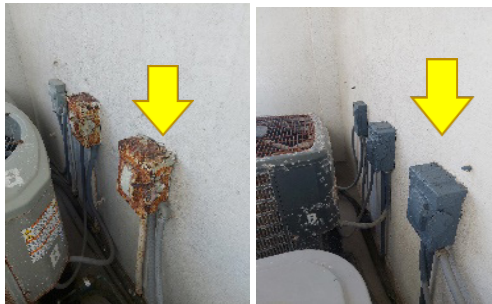
3 rd floor- before after
