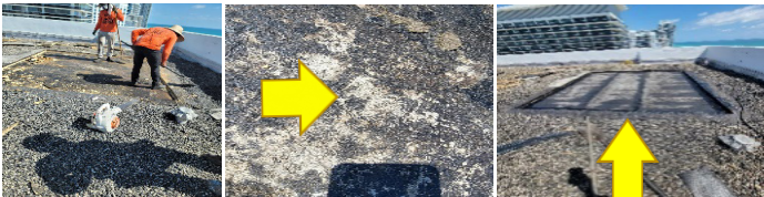
Hairline crack on the concrete
