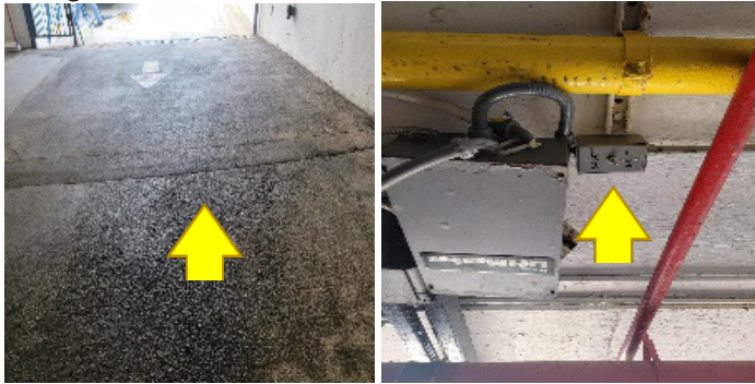
Garage floor sensor and switch.
