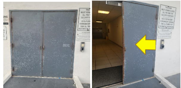
Contractor entrance (before)
