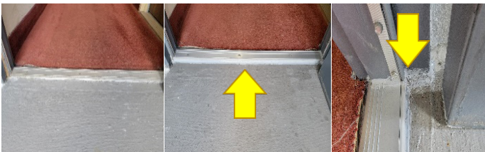
Before (11 th floor) after
