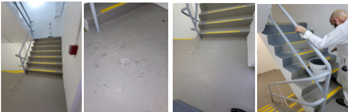
12 th floor before
