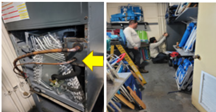
new coil installed
