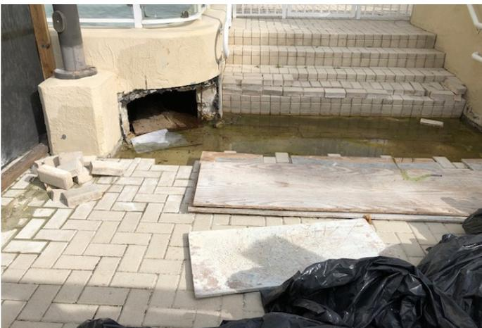
Waterproofing of SE corner of pool deck. Continuing water accumulation at this location has prevented completion of waterproofing of pool deck. The water is not pool water. Work is continuing to determine the source of the water.
