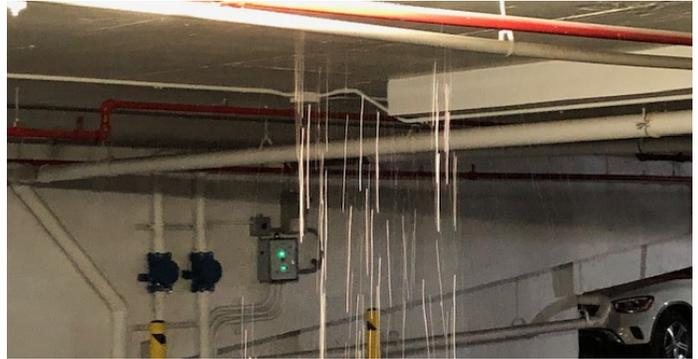
Basement Garage Ceiling Water Leaks. During recent rainstorm, several ceiling water leaks were observed in the basement garage. Investigation determined that the leaks occurred at concrete expansion joints that will be replaced as part of this project. Work is ongoing. Estimated project completion: March 2024.
