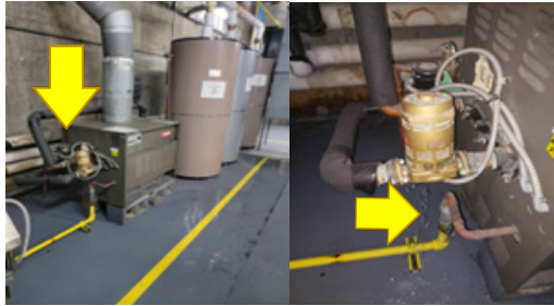
Leaking Pump
