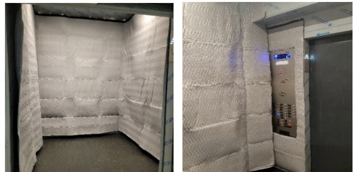
Service elevator – new wall pads
