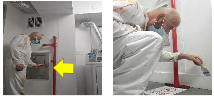
The fire sprinkler pipes were re-painted in red.
