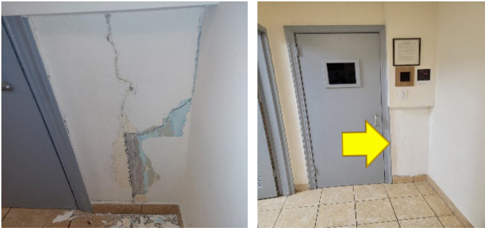
The entrance of the steam room (before & after)
