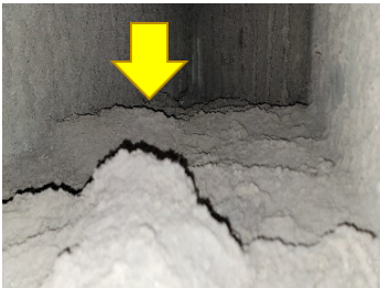
inside ductwork (before)
