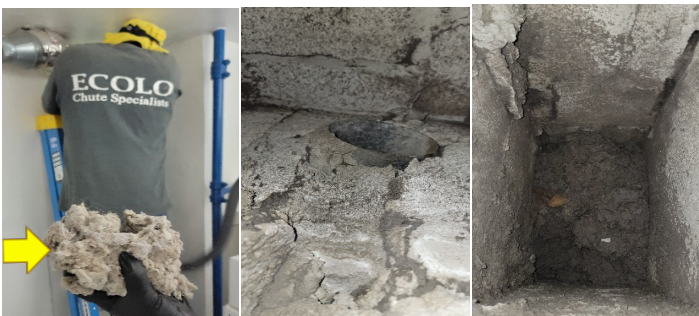
2 nd floor dryer vent into the shaft
