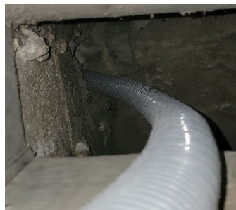
dryer vent exhaust pipe
