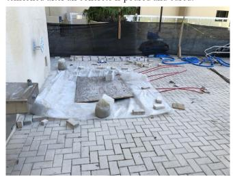
• Phases 4 and 5 (West Visitor Parking Lot) – Concrete surface and post tensioned cable repairs underway.
