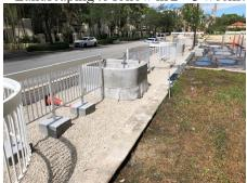
Phases 4 and 5 (West Visitor Parking Lot) – Removal of old surface coating is complete. Concrete surface repair is required prior to resurfacing. Repair method under development by Biller Reinhart.
