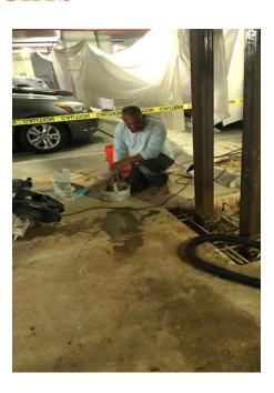
Pool Equipment Room door frame installed and grouted in. Door to be installed in May
