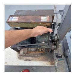
Put some lubricant on the chain that opens the parking garage door.
