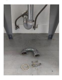
On the 11th floor, repairs were made to the water trap.
