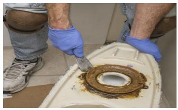
Your toilet's wax ring creates an airtight seal that prevents water and sewer gas from escaping. When the thick wax ring goes bad, you need to replace it right away to prevent leaks and damages to your neighbor's ceiling. Knowing the signs of wax ring failure will help you be proactive:
