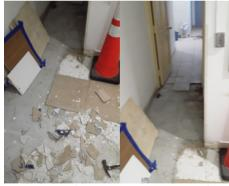
Mezzanine walls and marble floor holes, damaged by the removal of the old ADA lift, have all been patched and painted.
