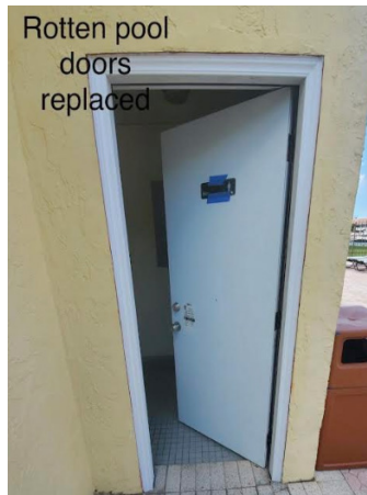
Rotten Pool bathroom door replaced
