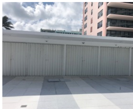
Old Cabana Doors being re-installed until the new ones are approved and produced
