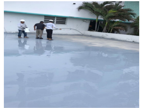
Parking deck waterproofing in progress
