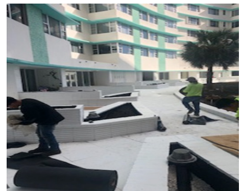
The landscape in front the Lanais is currently being installed by the Designer's team
