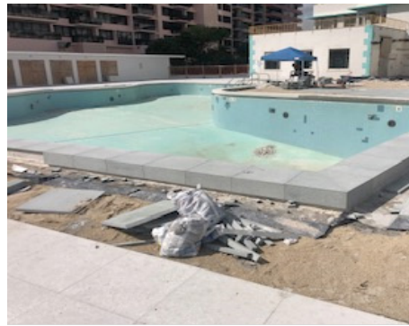
Pool coping currently being installed by the designated contractor
