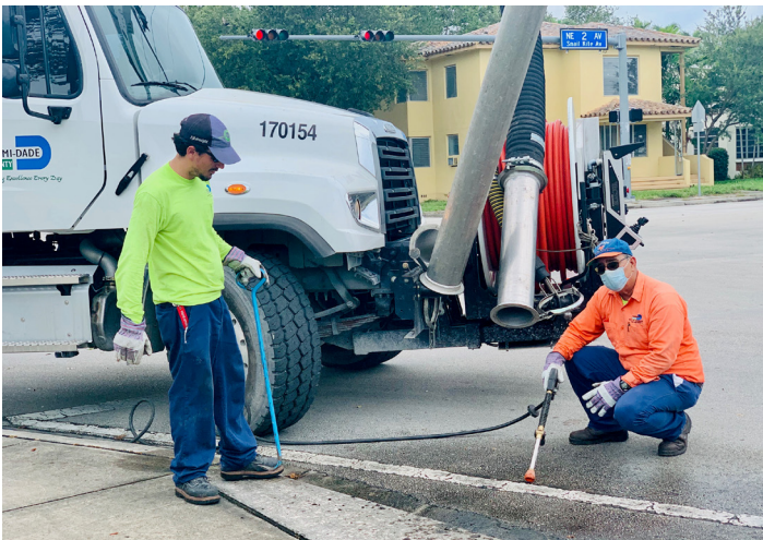
Working with Miami-Dade County to get our drainages clean.
