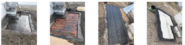
Remove roofing system to deck. Replace insulation and install new roof system
