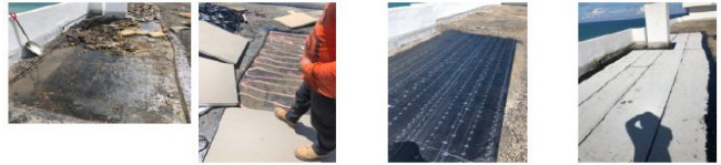
Remove roofing system to deck. Replace insulation and install new roof system
